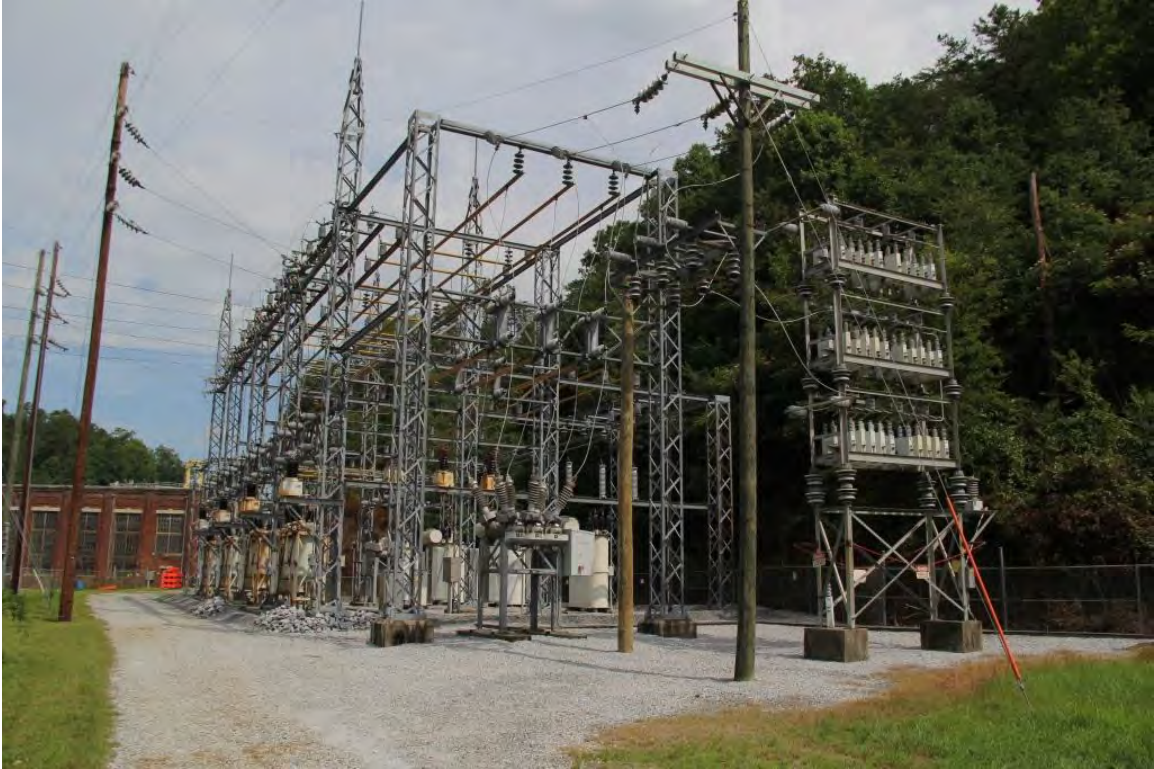
Substation, view to west
