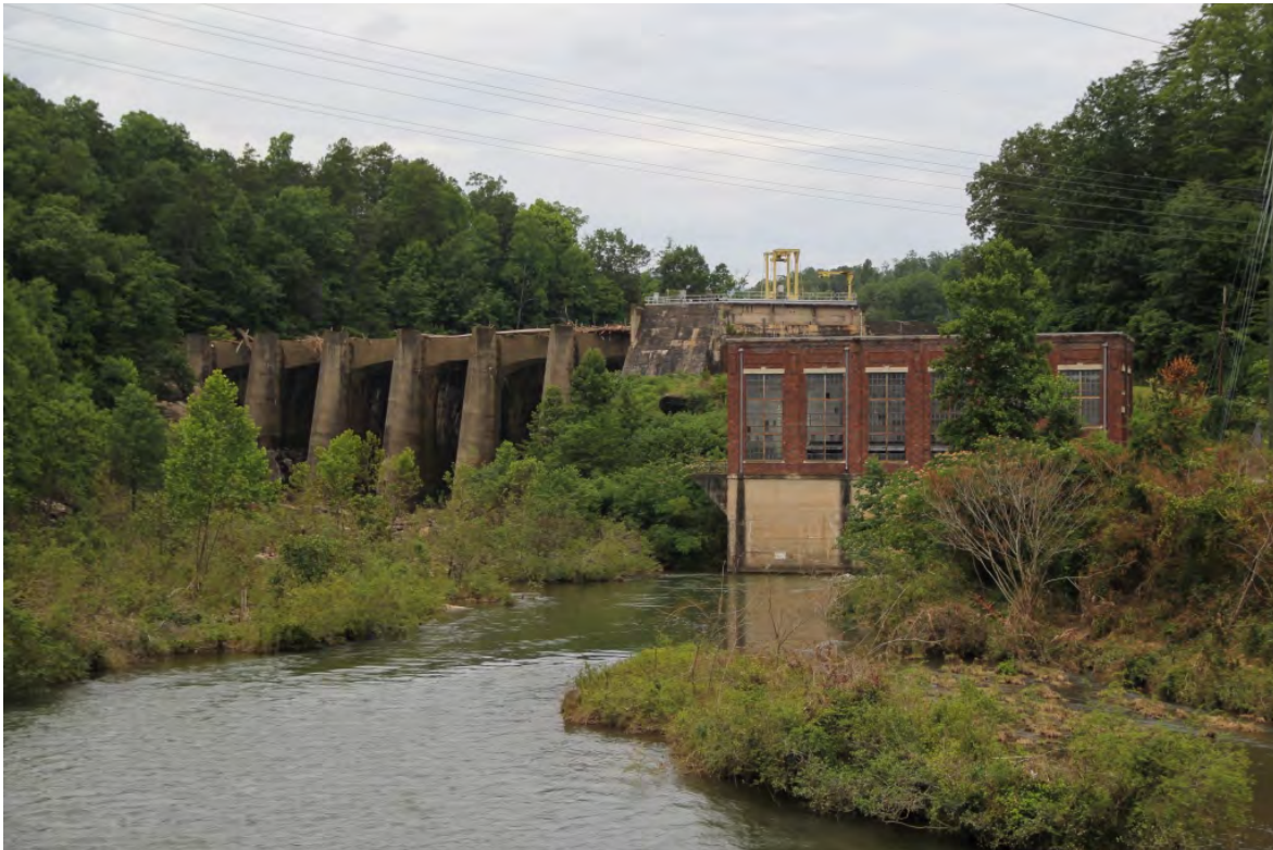
Turner Shoals Hydroelectric Station (PL 310), 3045 NC 9, overall view to northwest
