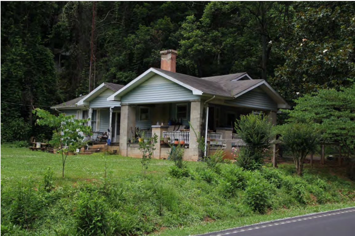
Operator's House, 3149 NC 9, oblique view to northwest [PIN P54-5]
