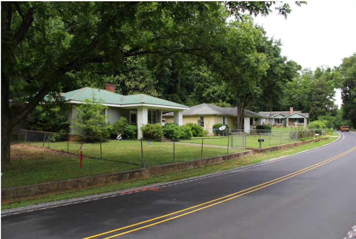
Operators' Houses, view to northwest along NC 9
