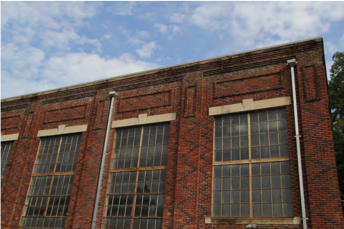
Powerhouse, east elevation (detail), view to west
