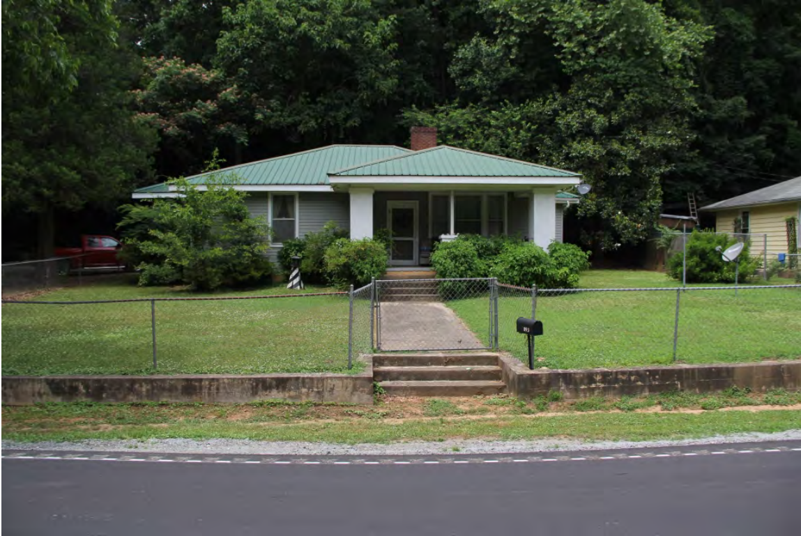
Operator's House, 3093 NC 9, façade, view to west [PIN P54-2]
