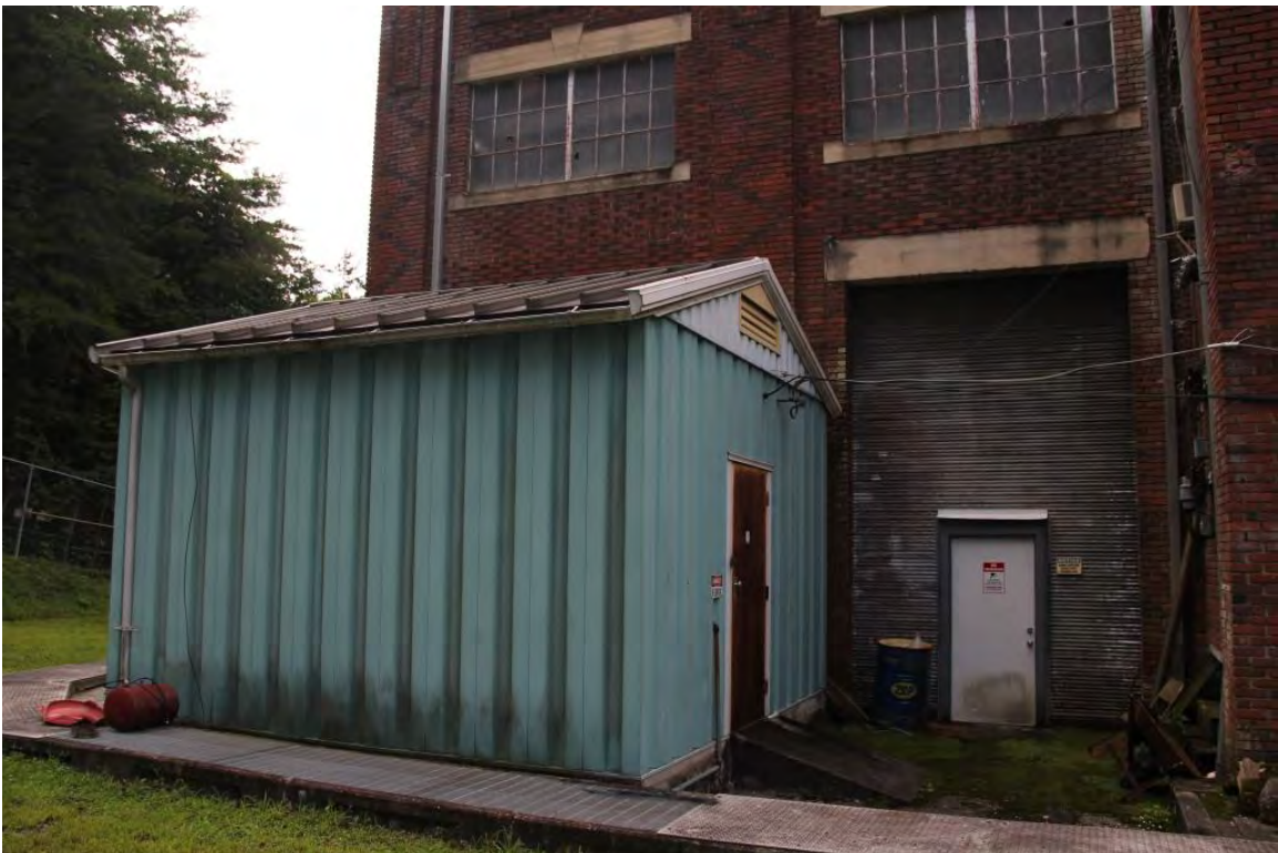
Powerhouse and storage building, view to southwest
