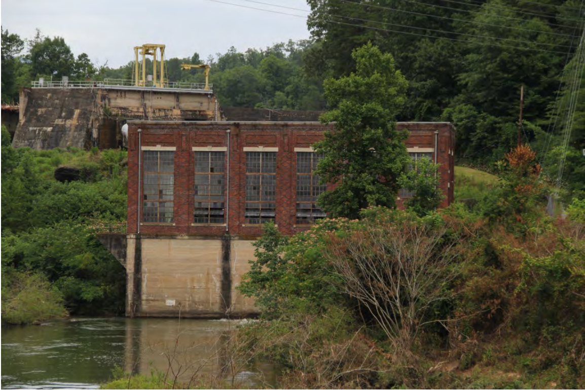
Powerhouse, view to west
