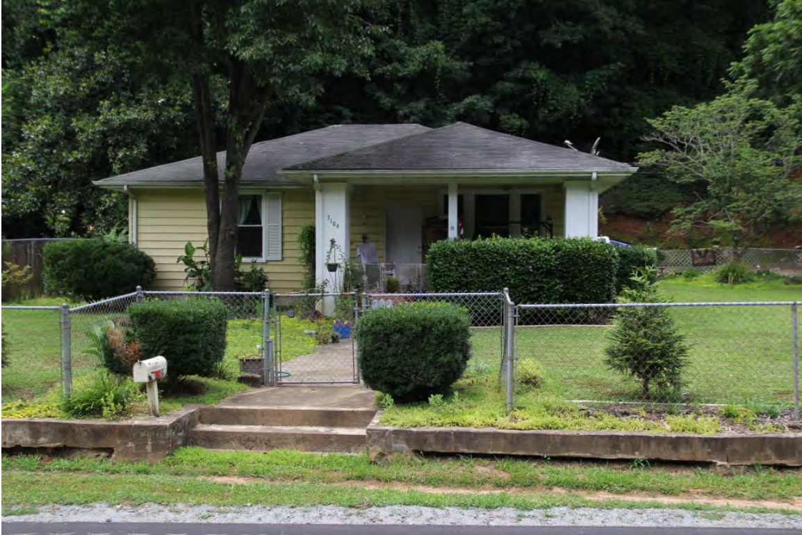
Operator's House, 3109 NC 9, façade, view to west [PIN P54-3]
