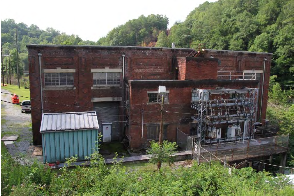
Powerhouse, rear elevation, view to southeast
