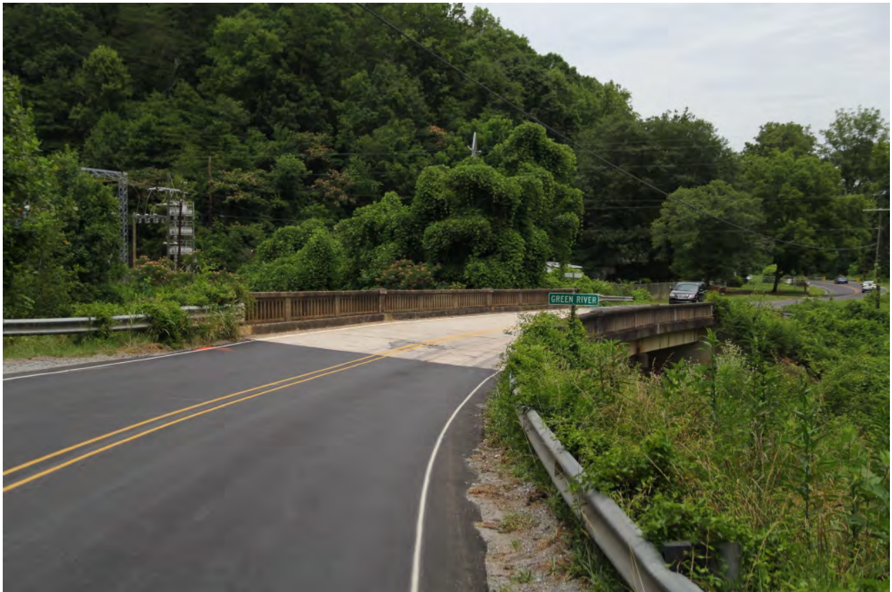
Turner's Bridge (Bridge No. 37), NC 9 over Green River, view to north
