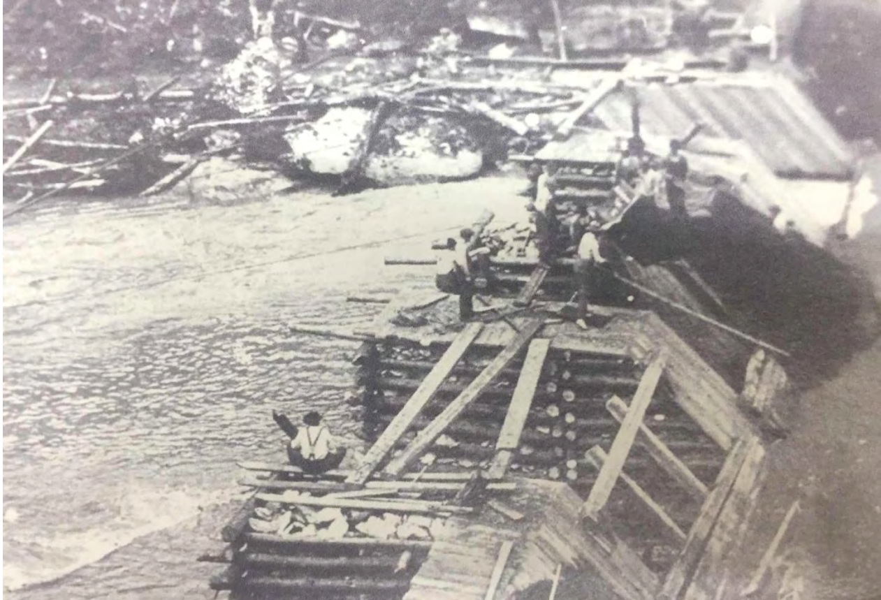
Lake Adger Dam construction, ca. 1923 [Collection of Polk County Historical Museum, 1999.1748]
