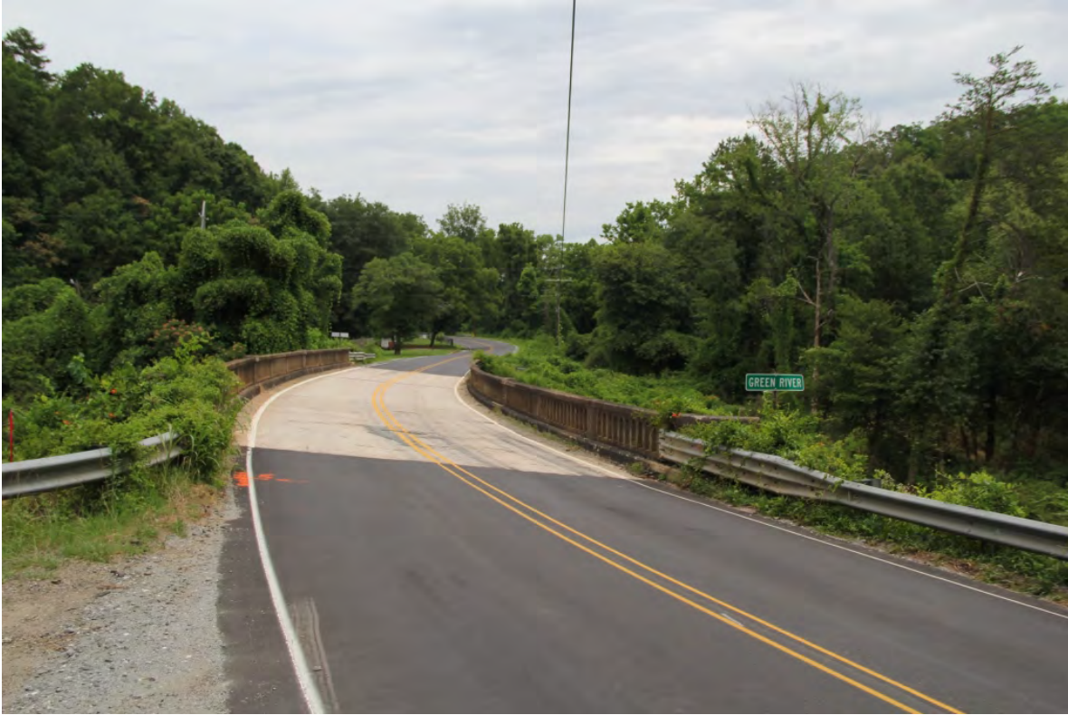
Turner's Bridge (Bridge No. 37), view to northeast along NC 9
