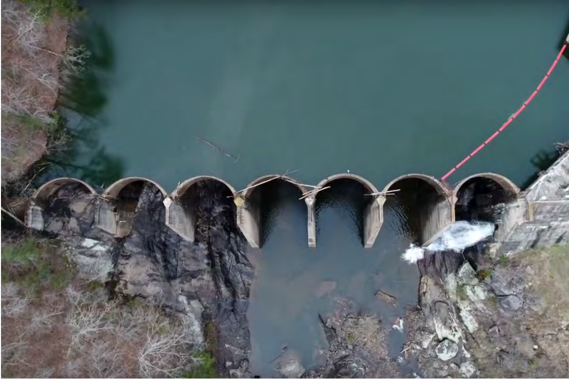
Turner Shoals Dam, overhead view (drone view by Toby Jenkins, March 22, 2017)
