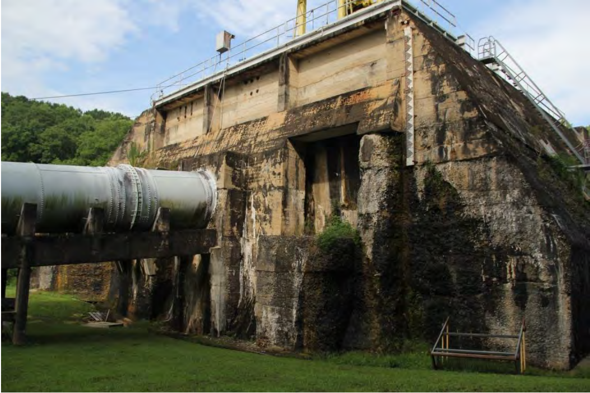
Intake structure, view to southwest
