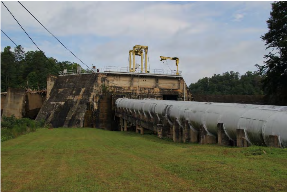
Intake structure and penstocks, view to west
