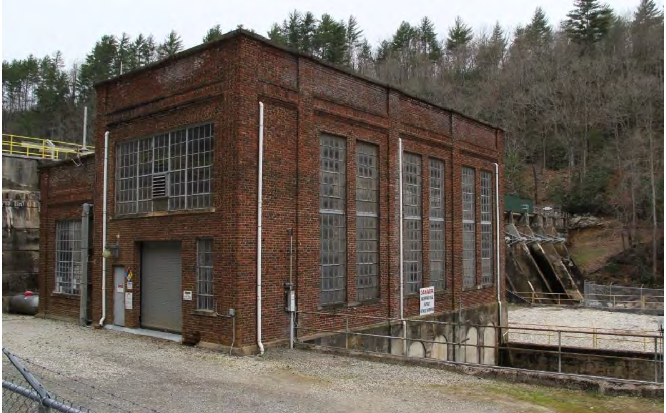
Mission Hydroelectric Plant (CY 54), 1924, oblique view to southeast
