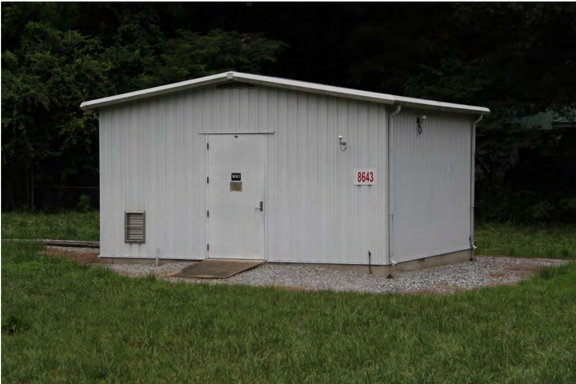
Utility building, view to north
