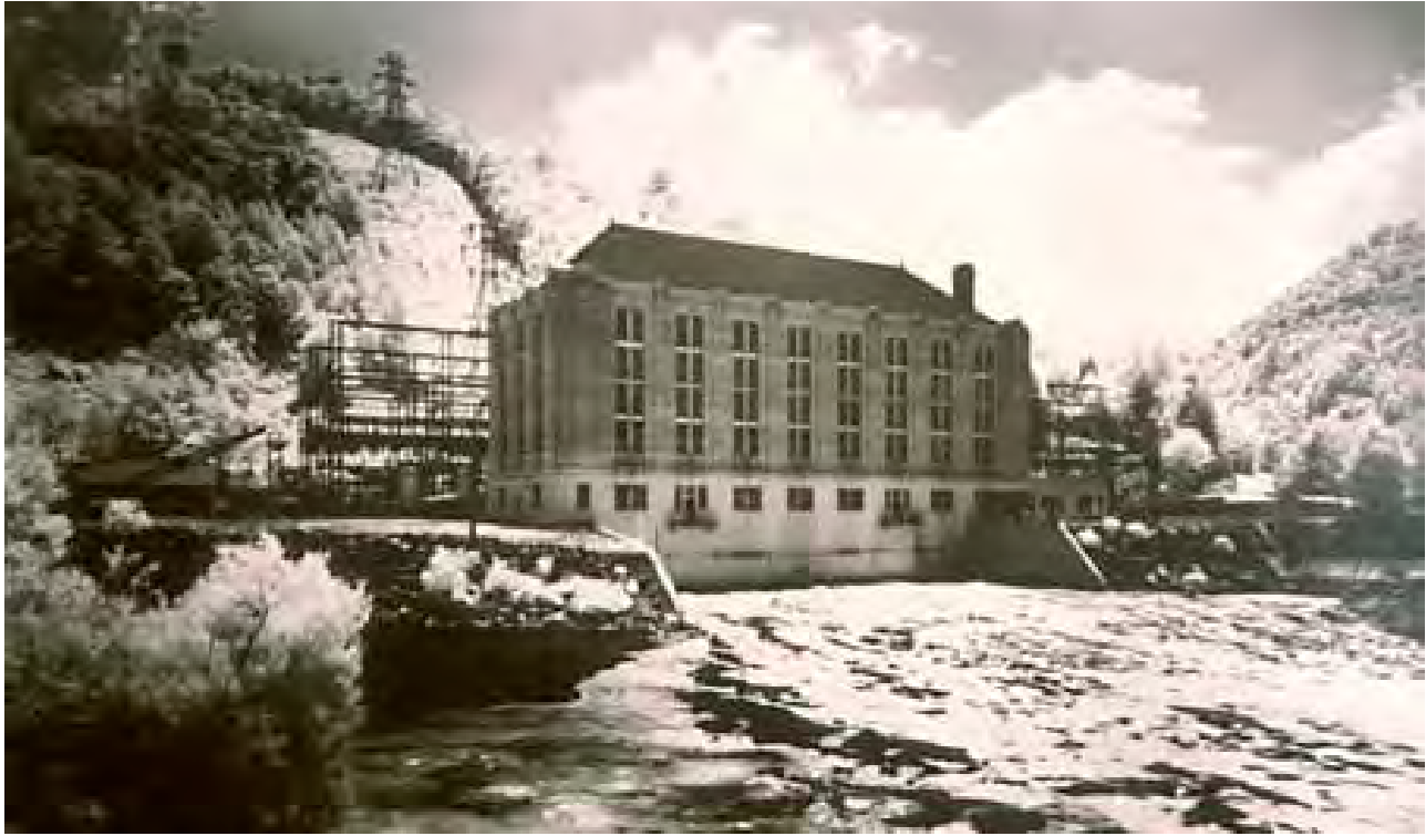
Walters Hydroelectric Plant (HW 268), September 1947 [North Carolina Collection, K275-S, Pack Memorial Library]
