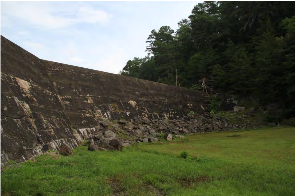
Containment wall (extension of Turner Shoals Dam), view to north
