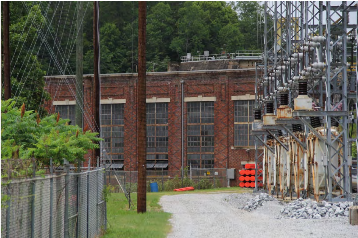
Powerhouse, view to southwest
