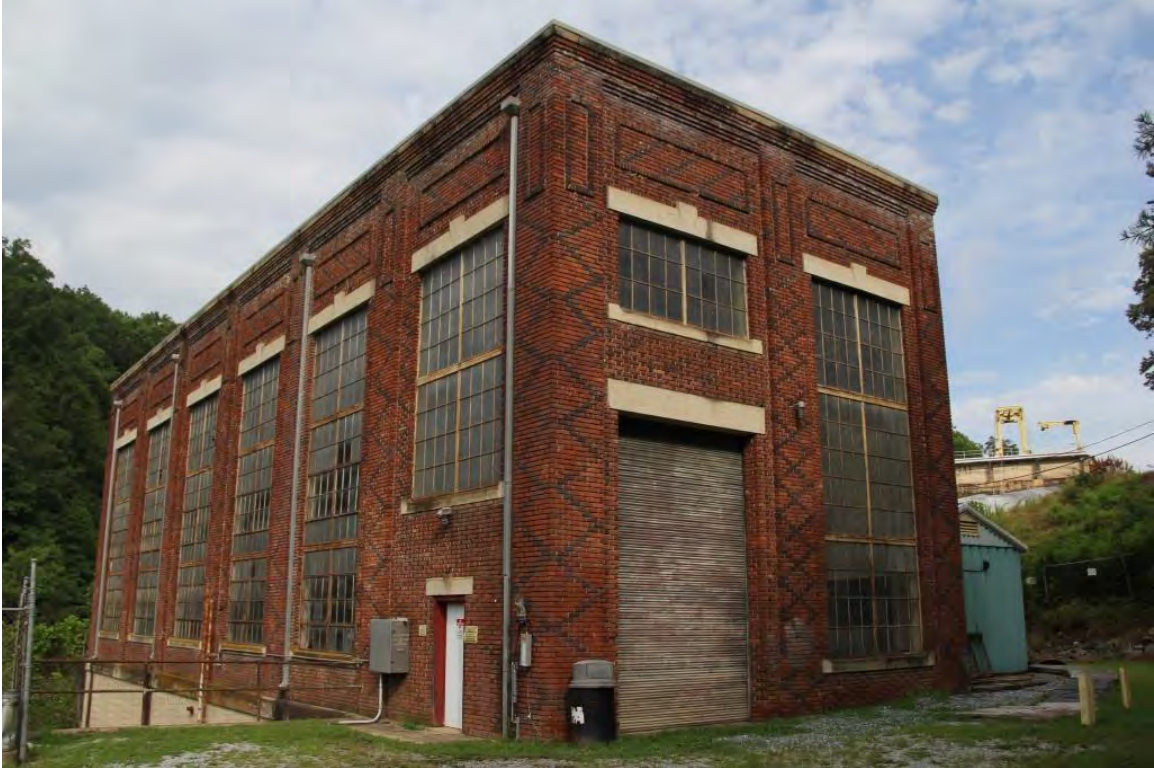
Powerhouse, oblique view to southwest
