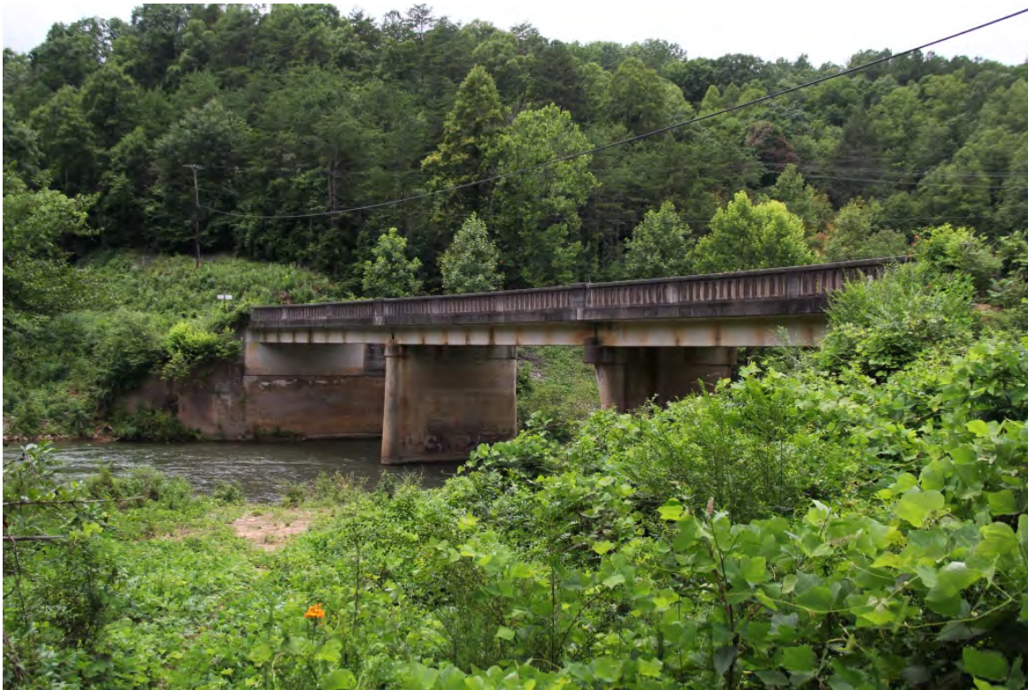
Turner's Bridge, view to southwest
