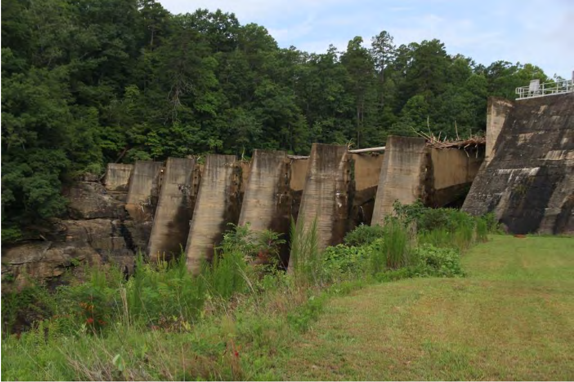
Turner Shoals Dam, overall view to southwest
